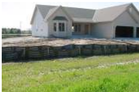
Above: Proper silt fence installation
