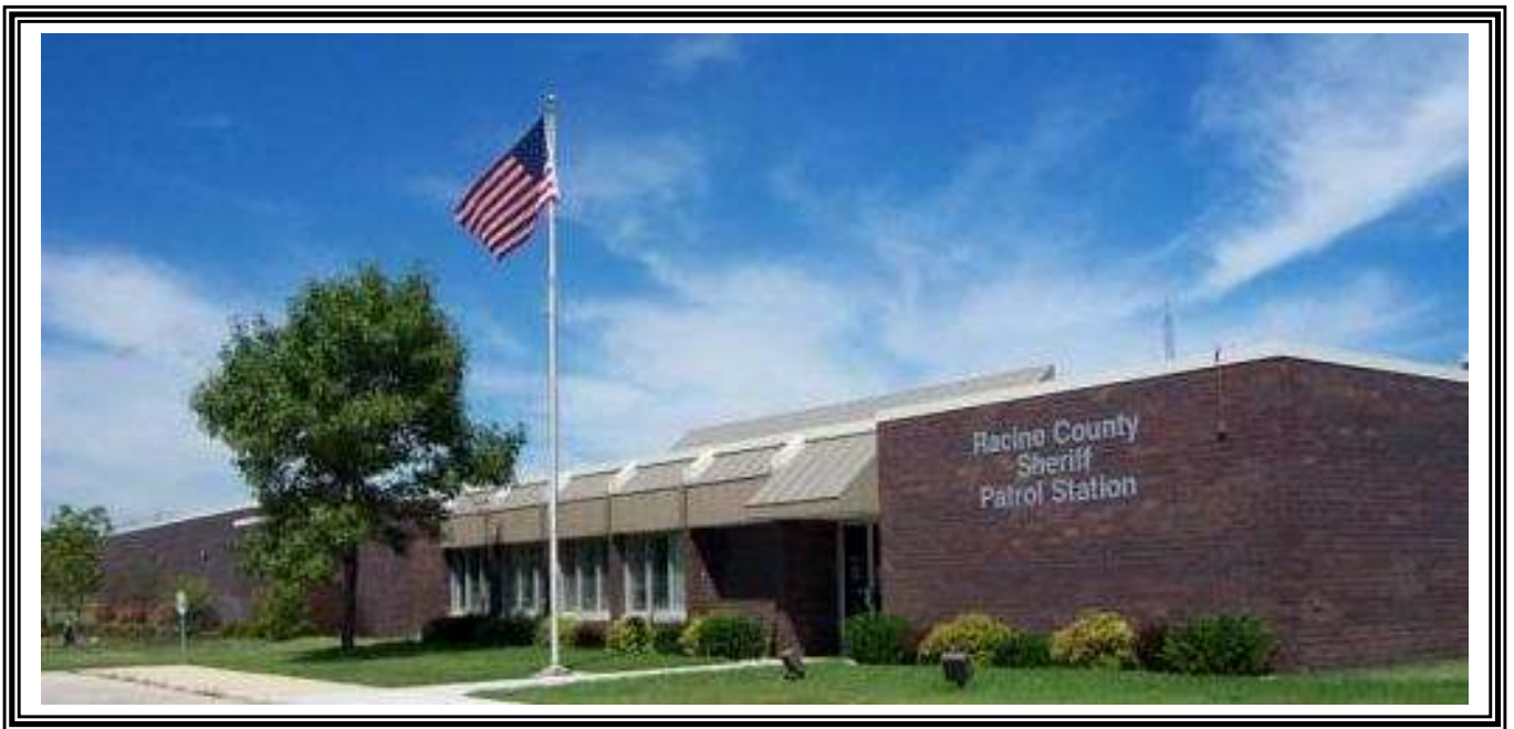
Racine County Communications Center & Patrol Station
