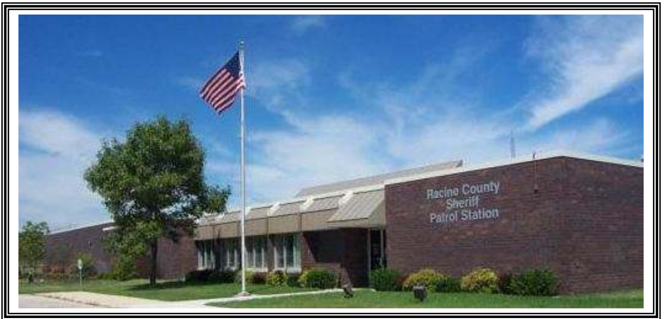
Racine County Communications Center & Patrol Station
